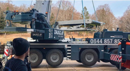
Treadmill is unpacked and brought in by crane.
