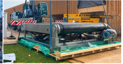
Treadmill is unpacked and brought in by crane.
