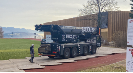
Special heavy-duty crane needed for installation
